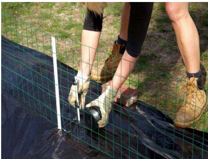
Step 8: Stringing the first row of fence wire
