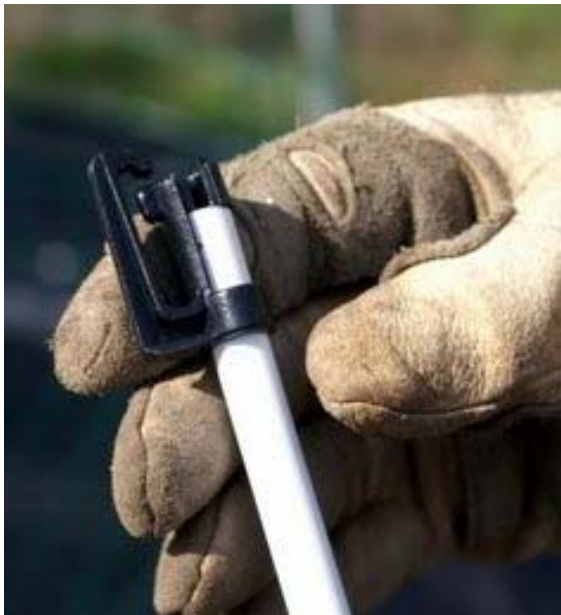
Step 5: Sliding on the insulator
