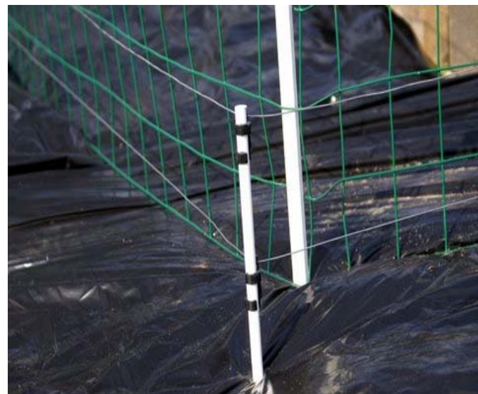
Both wires strung. The fence is finished and awaiting an energizer.
