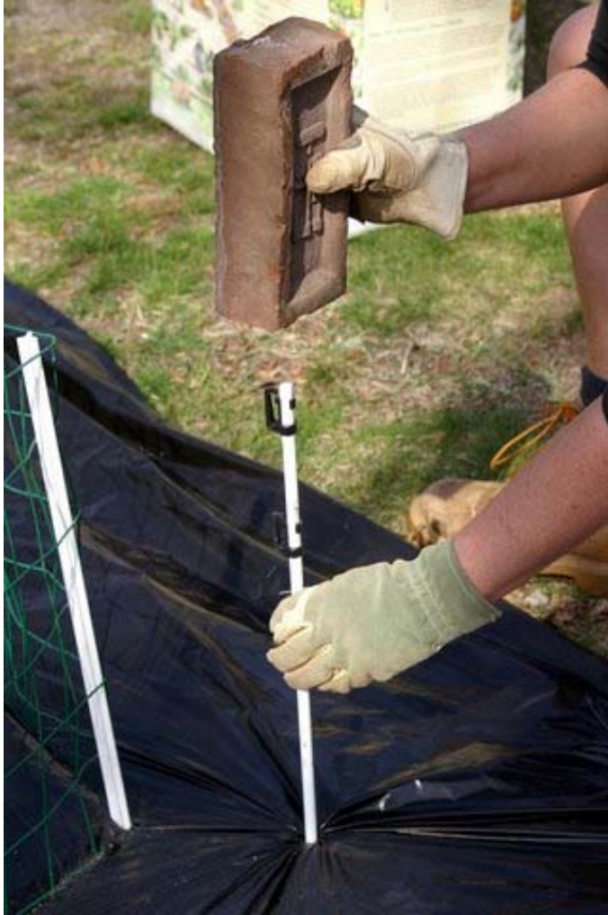
Step 7: Inserting the corner 18" post to a depth of 9"
