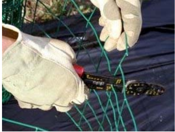
Step 4: Cutting the barrier fence to fit.
