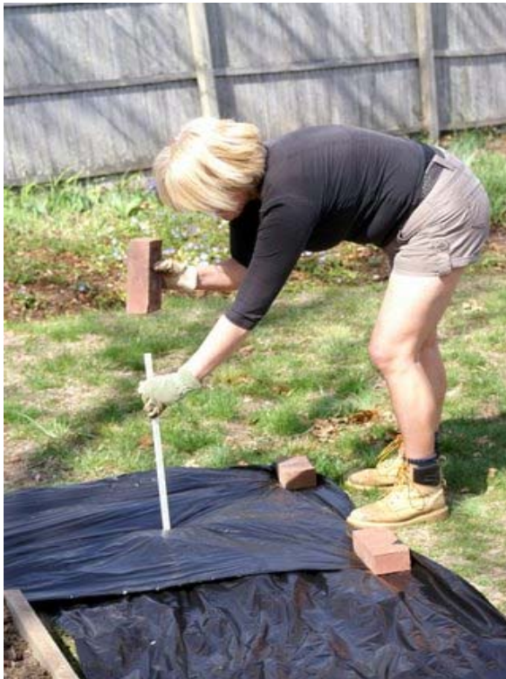
Step 2: Inserting the 27" fiberglass posts into the ground.
